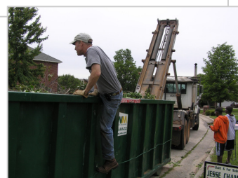
Chris Hulen smashing down the last load of debris.
